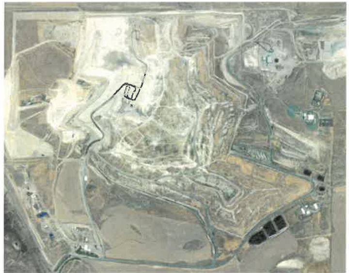
Figure 8-1. Roosevelt Regional Landfill Aerial View.
